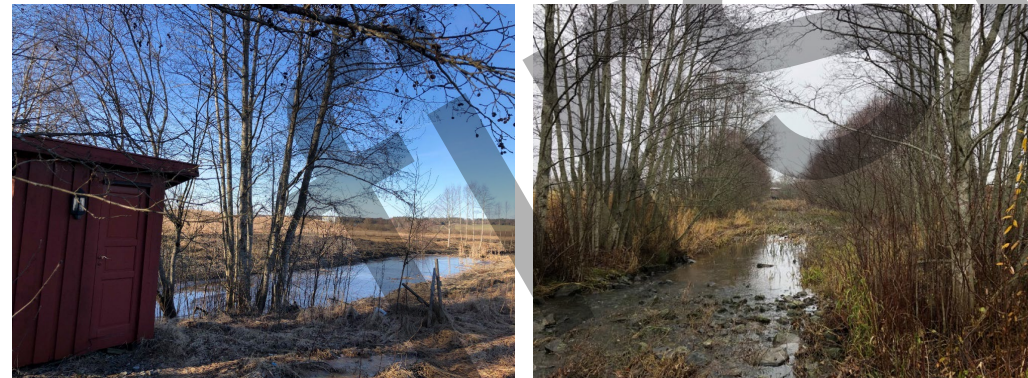
Skuterud CW: sedimentation pond and measuring station (left) and first vegetation filter (right). Photos by A-G.B.Blankenberg.
